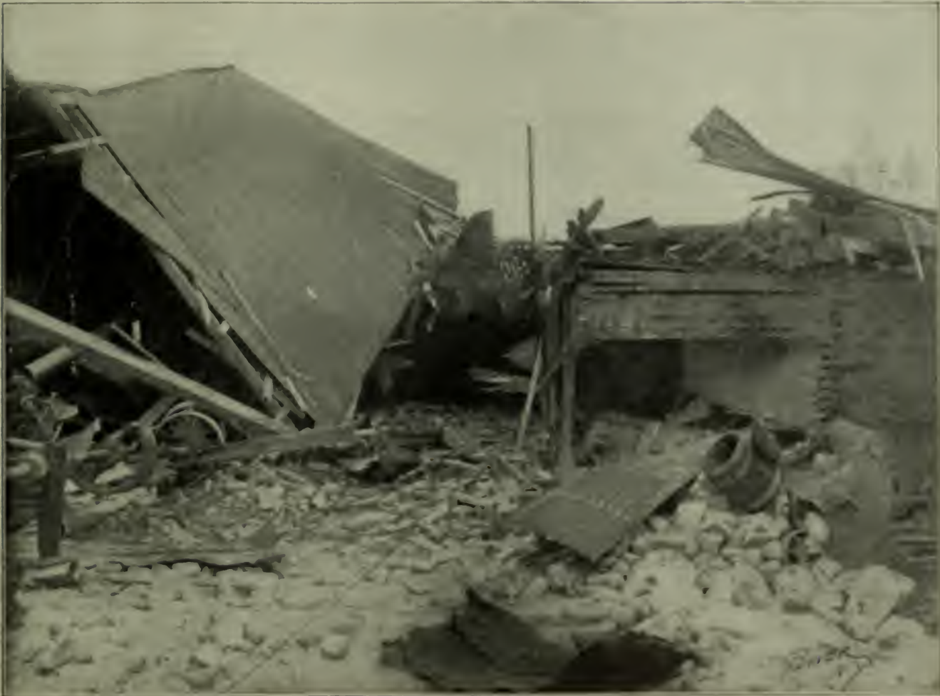
BOILER EXPLOSION AT DOWAGIAC, MICH.
